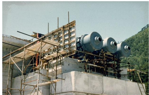
Fig. 17: Application of the hysteretic dampers to the bridge Fella of the Udine-Tarvisio Motorway
