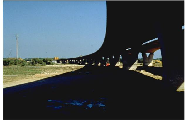
Fig. 20: The Coltano Viaduct, 10 km long, is the largest application of the base isolation in the world
