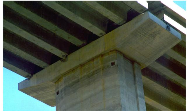
Fig. 26: Detail of the beams supports after 1 meter displacement
