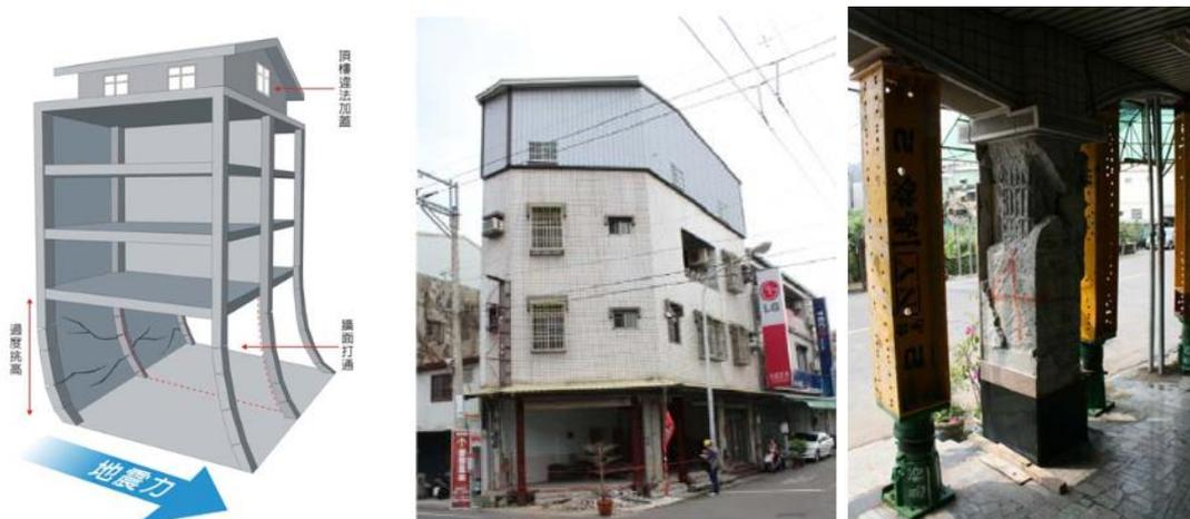
Illustration 10.2-1. Exemple de construction avec un rez de chaussée souple. Source: Seismic preliminary evaluation of low-rise residential buildings in Taiwan, Tsung-Chih Chiou, Yaw-Shen Tu, Wen-Cheng Shen, Pu-Weng Weng, Shyh-Jiann Hwang, Lap-Loi Chung, NCREE 2016
